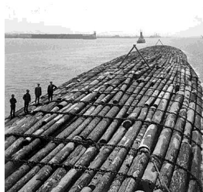
Figure 10 – Benson Log Rafts
